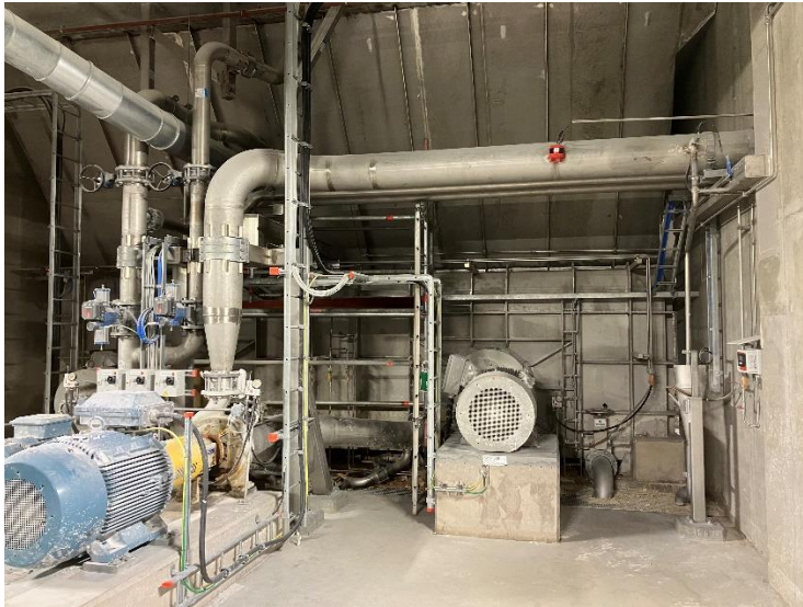
Figure 2: ACT-2500, Ampliforce™ consistency transmitter installed on broke line
